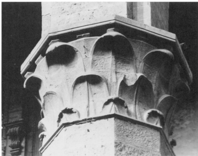
Fig. 16. S. Croce, Florence, begun 1294–95, interior. The leafwork in the S. Croce capitals, which adheres closely to the calathus, contrasts with the much more three-dimensional treatment of the leaf forms in the Orvieto capitals. (Author)
